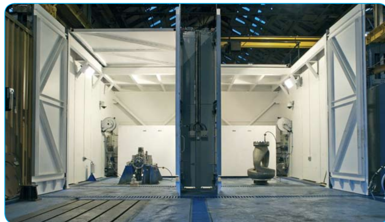
• 2 High Pressure test booths with doors open & one roof retracted
