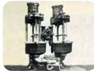
First manufacturing order of two BFPs taken in 1893, installed in RMS Campania by the Fairfield company
